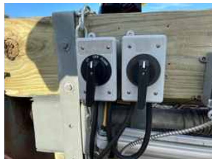
Boat lift switches, one side at a time (reversed: UP = down)
